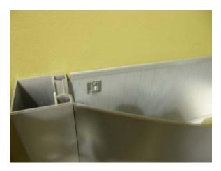
(1) Hang the Serene Water Feature on the Wall Bracket. Use the clips on the bracket and the square holes on the water feature. Push down gently until the water feature in snug on the clips and hanging level.
